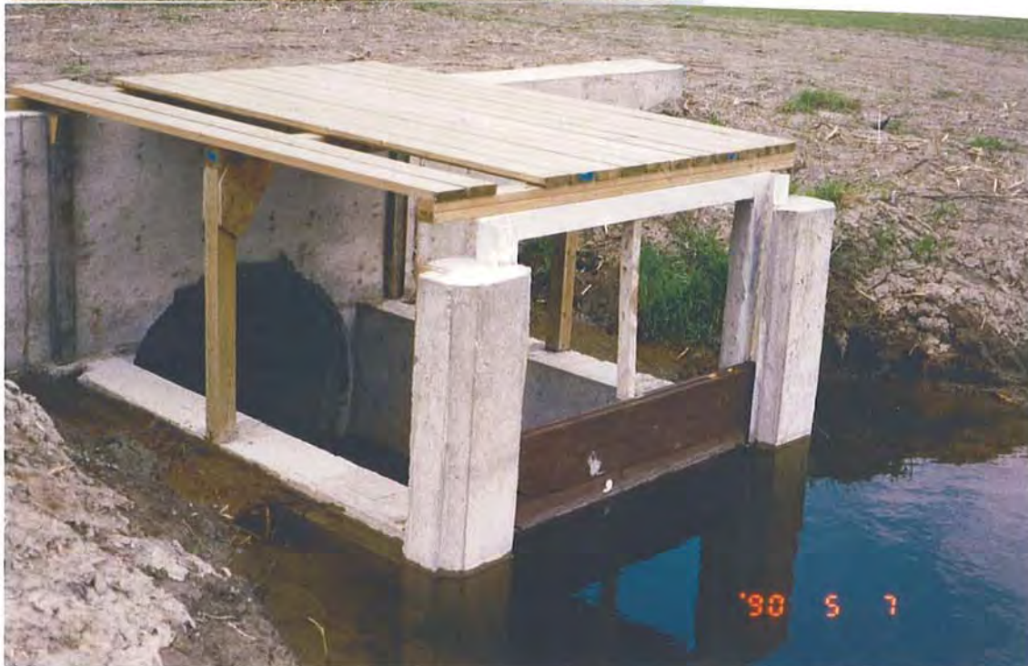
A water level control structure on a municipal watercourse near St-Robert, Richelieu County, Quebec. Flashboards are added and removed on front and sides to adjust the water level.
